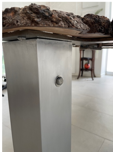
Figure 12. Insert to leg bolt
